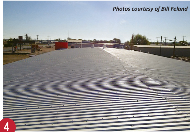
Metal roof after Rapid Roof® acrylic top-coat.
