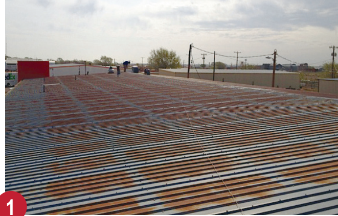
Rusty metal roof prior to restoration work.
